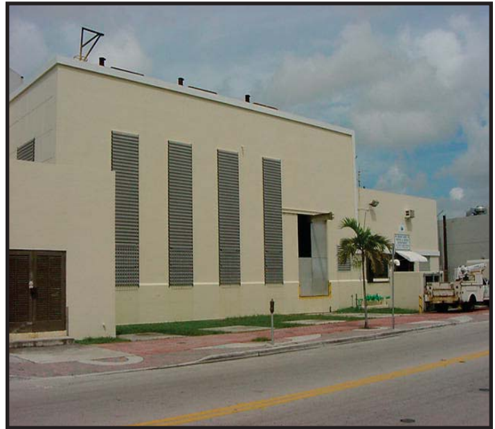
Pump Station No. 1 today
