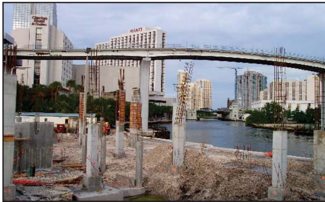
One Riverview Square under construction (2)
