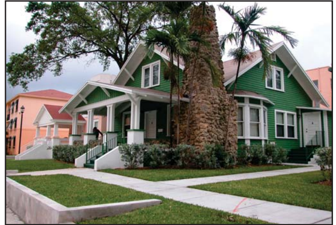
A recently restored wood frame house in the Lummus Park Neighborhood
