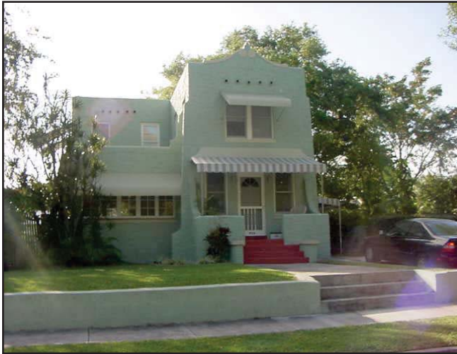
Two-story masonry house in Spring Garden
