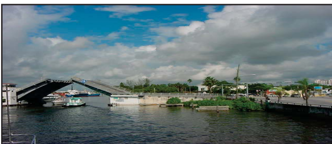
5th Street Bridge (18)
