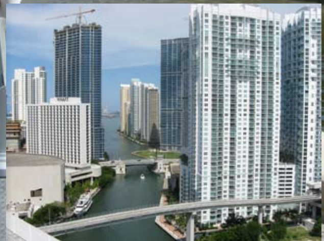
Viewed from the riverwalk, dredging nears completion at the mouth of the Miami River.
