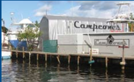
New Campeones Boatyard and Marina at 600 NW Seventh Avenue on the Seybold Canal
